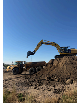
Obtaining a gradation sample
